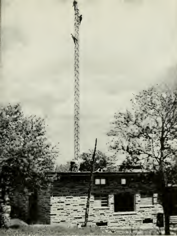
Workmen rig a temporary television antenna atop the transmitter building of CBFT, Montreal.
