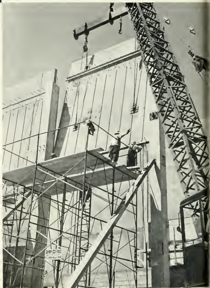
A huge crane swings a 16-ton concrete panel into place as part of the studio's outer wall.
